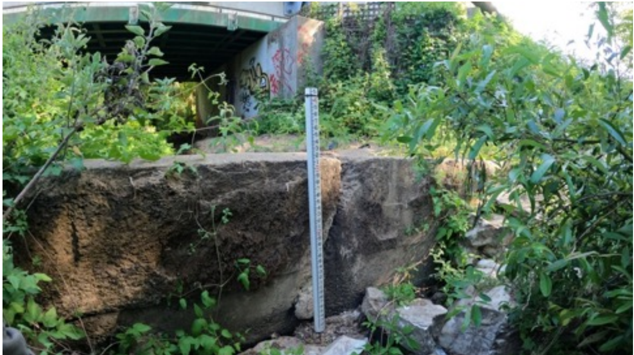
Figure 47. The barrier downstream of the Old Stage Road crossing (SRC). The height of the retaining wall was approximately 0.98 m (3.2 feet). Flows sufficient to allow for passage over this structure were not observed during 2020 or 2021 sampling (see Figure 19 for an overhead view during a period of flow).
