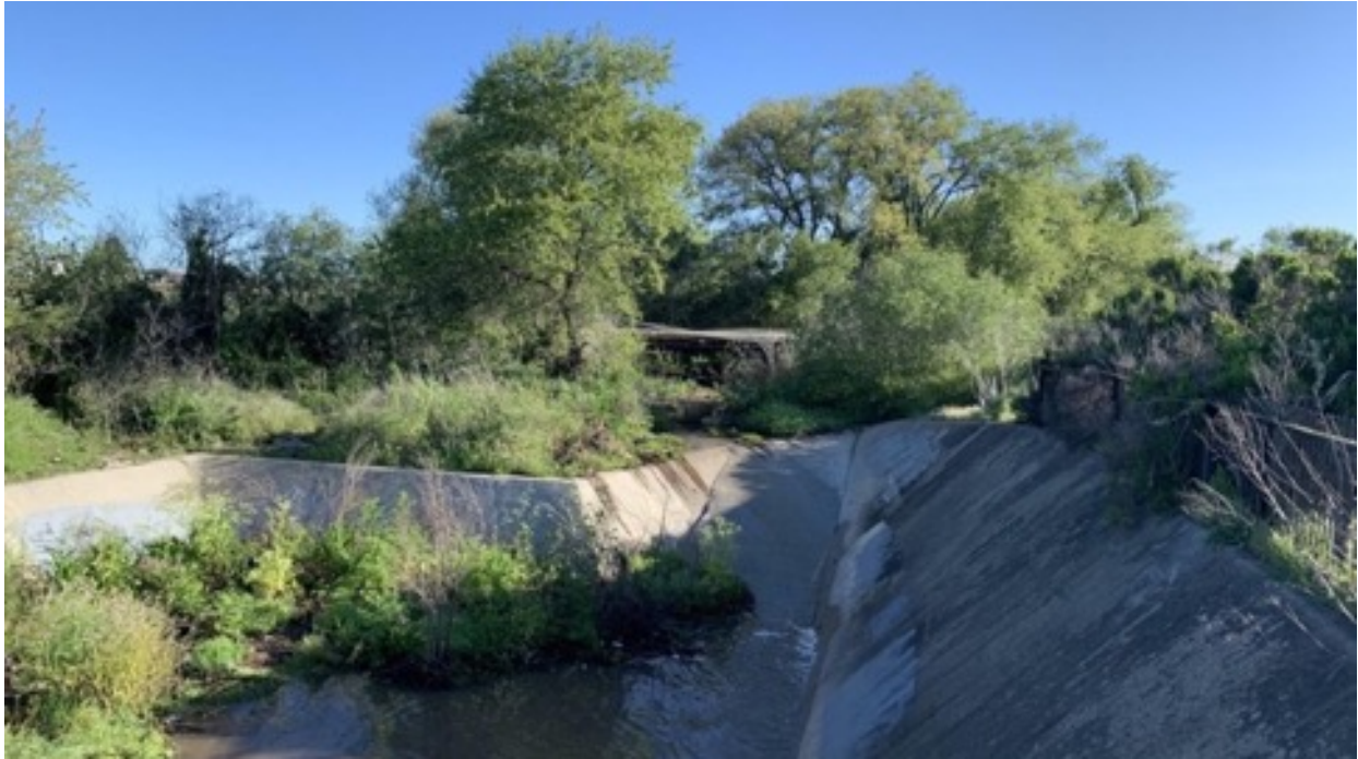
Figure 10. The large concrete barrier located just north of the Boronda Road crossing on Gabilan Creek. Photo was taken on April 7, 2020, 24 hours after a large precipitation event. Laminar flow down the concrete ramp suggests this barrier may have remained impassable at all but the highest flows experienced in 2020.
