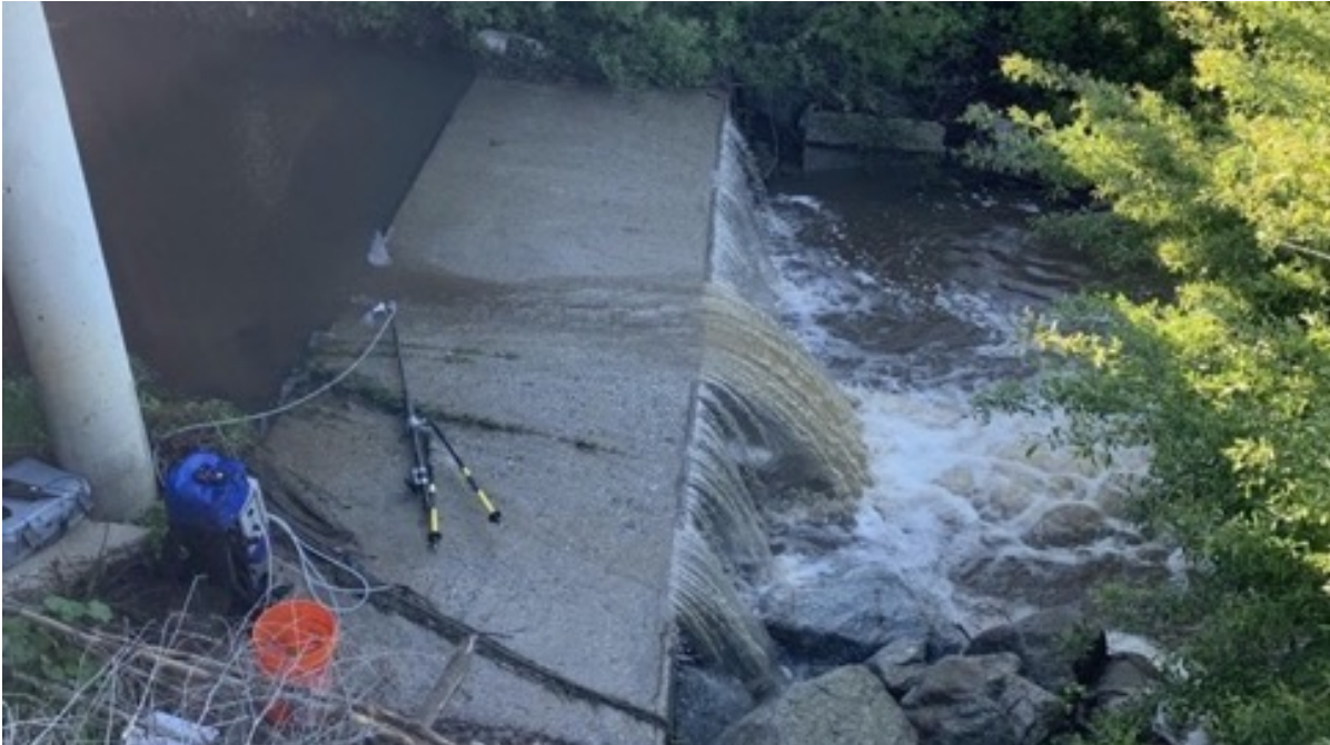
Figure 6. The sampling site located at the Hebert Road crossing (HEB). The height from the top of the barrier to the substrate below was 1.22 meters (four feet), as measured during a period of no flow. Photo taken April 7, 2020.
